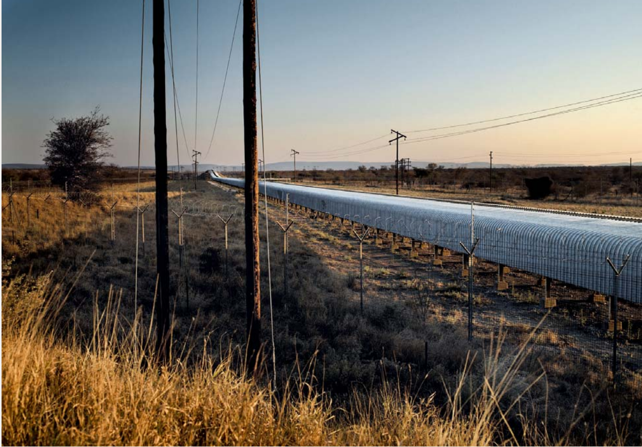
A conveyor carrying coal from Grootegeluk mine to Eskom's Matimba power station near Lephalale, Limpopo
