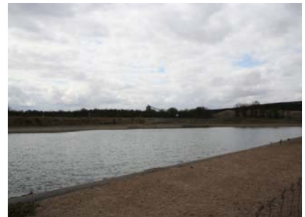
Return water dam - Tshikondeni co-disposal facility
