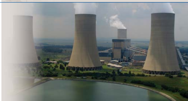
Lethabo power station in Vereeniging.
