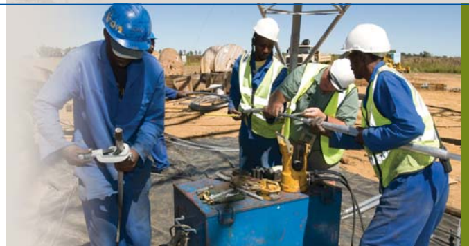
Major transmission line construction strengthens the national grid.
