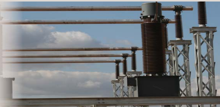
Top: Construction of Medupi power station is advancing well. Bottom: Insulators in the new 132kV yard at Medupi.
