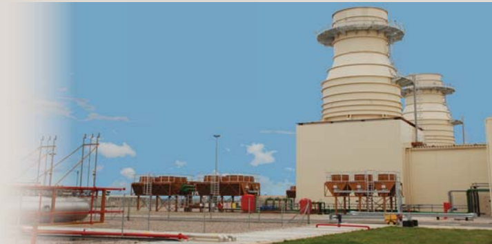
The Goukwa open-cycle gas turbine station near Mossel Bay.
