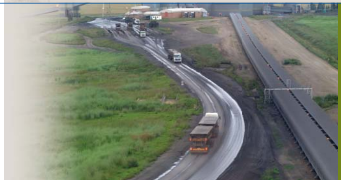
Coal trucks offloading at the Majuba power station stockyard.
