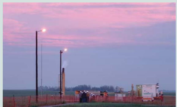
Eskom's underground coal gasification demonstration plant in the foreground.
