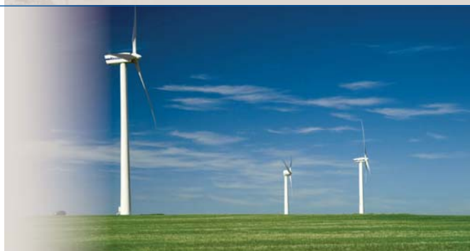
Eskom's Klipheuwel wind farm near Bellville.
