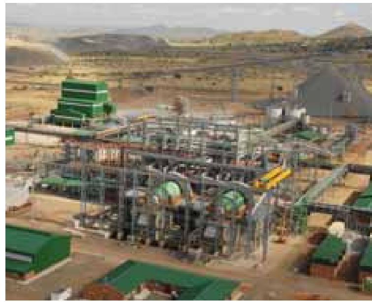
PP Rust Potgietersrust
