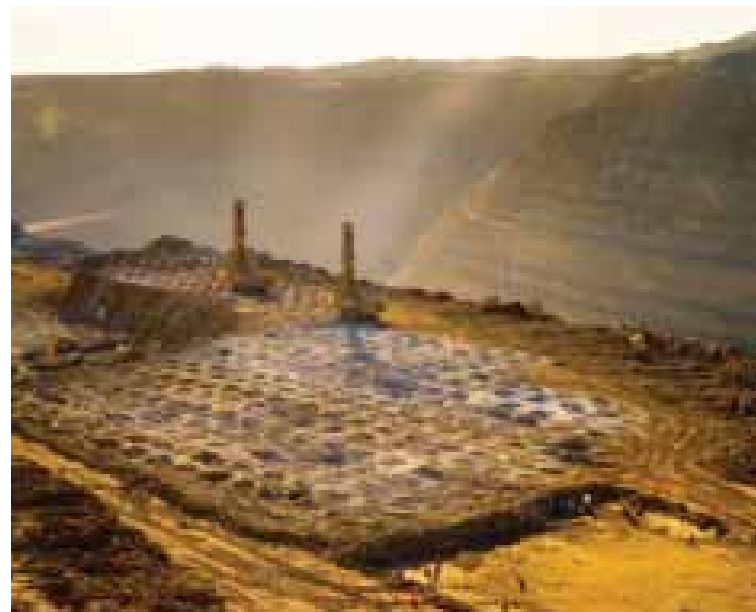
Drilling and blasting operations at Rössing Mine
